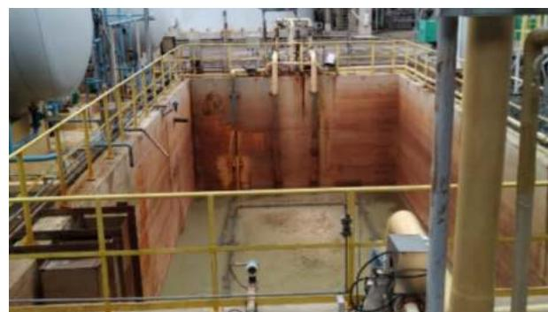
**Gambar 4.5** Neutralizing Pond
